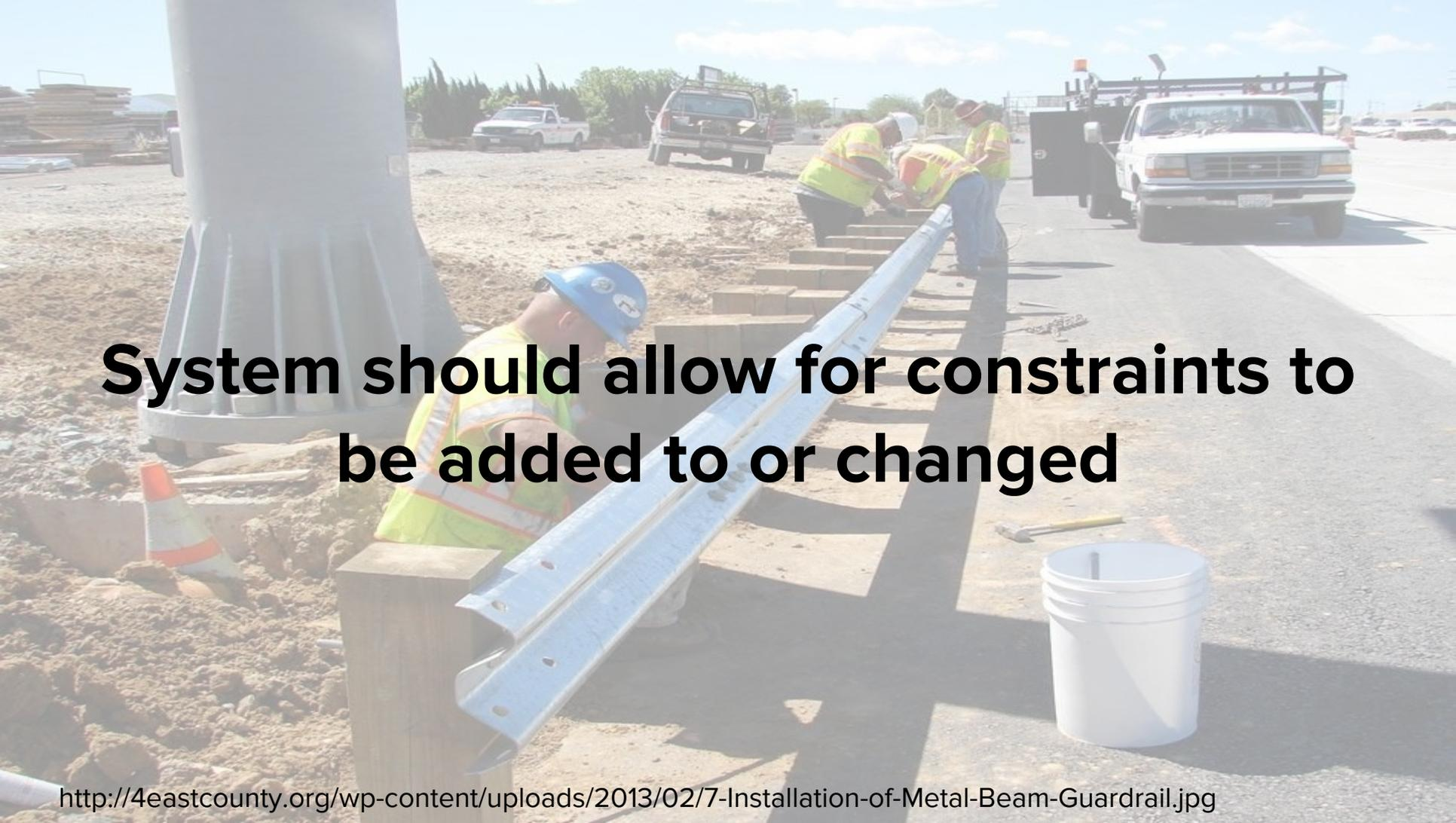
A photograph showing construction workers in high-visibility vests and hard hats installing a metal beam guardrail on a road shoulder. The guardrail is being placed on concrete blocks. In the background, there are several pickup trucks and a large utility pole. The scene is outdoors on a sunny day.
